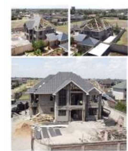
Membry project. Scope of work: Design and build. CONTRACT VALUE KSH 45,000,000
