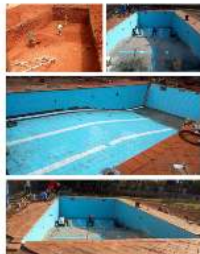
Nyeri Baptist Academy. Scope of work: Swimming pool construction.
