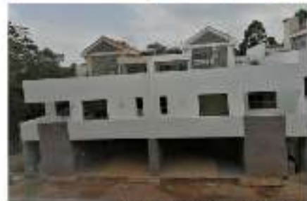
Muthaiga town houses on Nivasha lane. Scope of work: Fit-out.
