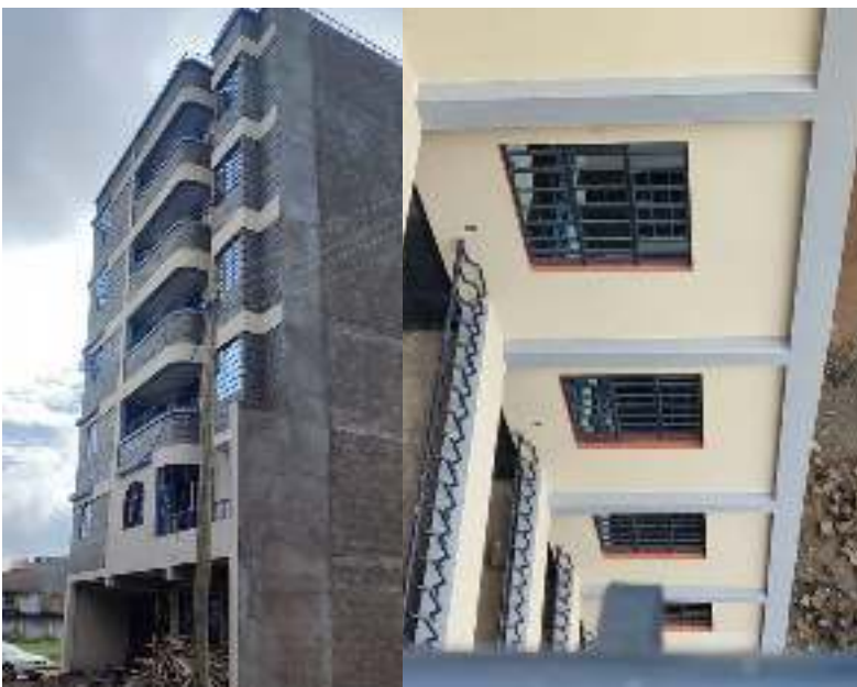
Umoja 3 Residential Apartment CONTRACT VALUE KSH 25,000,000
