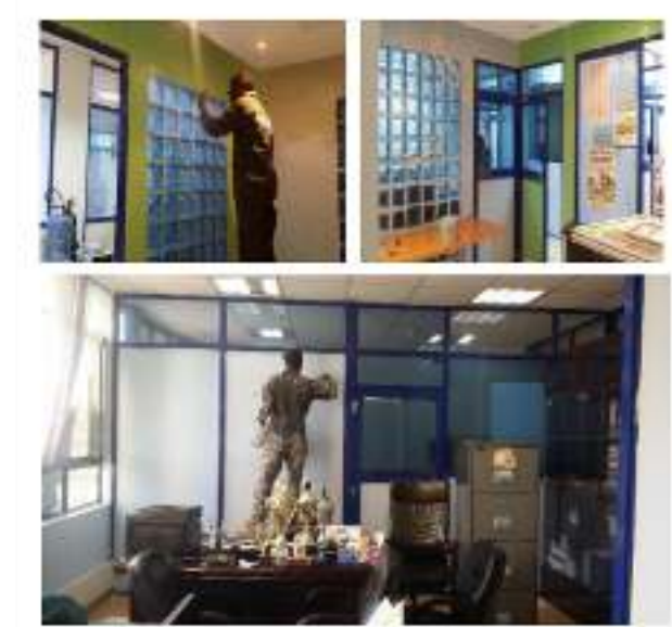
Athi Water offices in upperhill. Scope of work: Paintworks CONTRACT VALUE KSH 300,000
